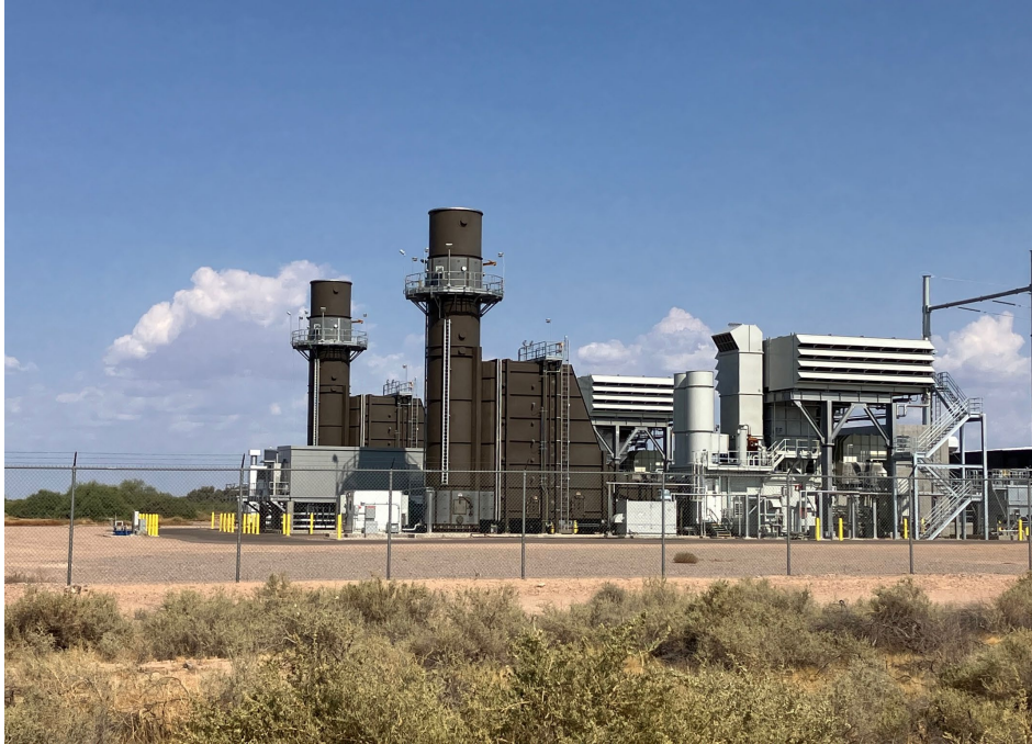
Source: GE LM6000 Units at Desert Basin in Casa Grande (SRP)
